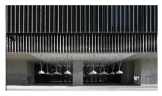
The M+ façade is made up of 140,000 pieces of ceramic tile laid out in a horizontal louvre structure to contribute to shading the interior. The modular terracotta cladding also extends to the podium and some sections of the ground floor and references traditional Chinese roofs. The tiles were made from clay in a ceramic factory in Chianti, Italy, assembled in precast units in Shenzhen and then shipped to Hong Kong.
