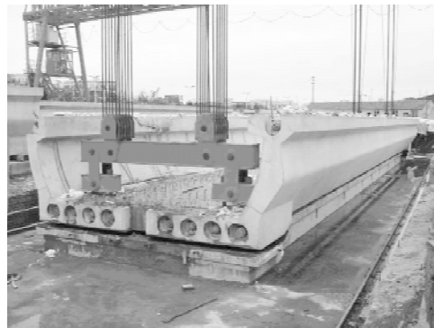
Figure 4 Cross section of U-shaped girder.
