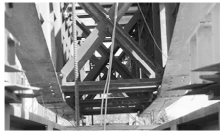
(b) truss transverse bracings
