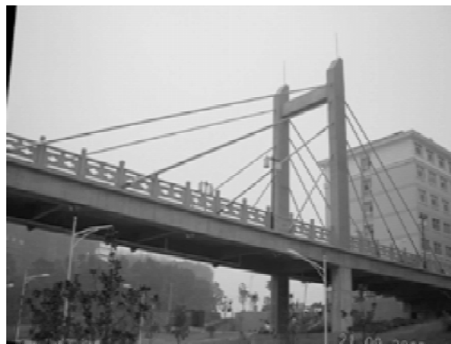
Figure 14 China's first high-performance CFRP cable stayed bridge
