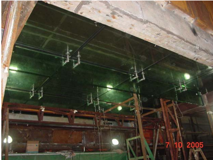
Figure 5: Glass Roof Specimen The glass is used as structural elements as glass beam.
