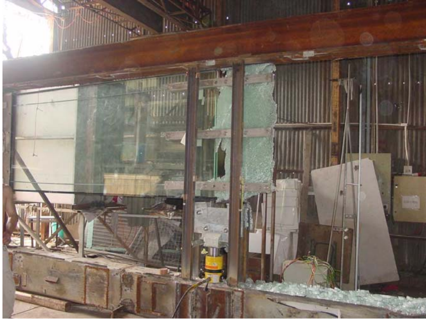
Figure 19: Specimen tested to failure
