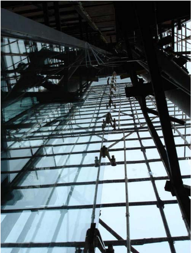
Figure 17: View from inside
