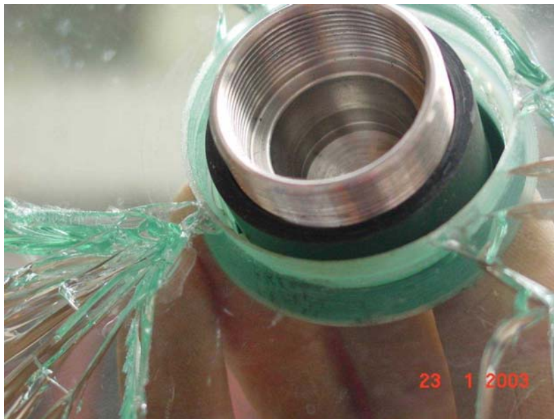
Figure 15: Closer look at the fixings
