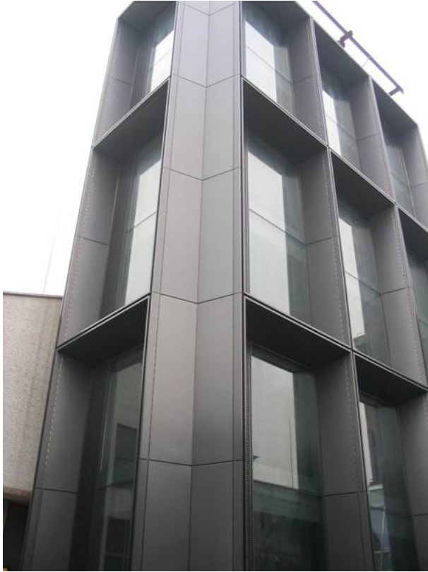
Figure 1: Curtain Wall Specimen
