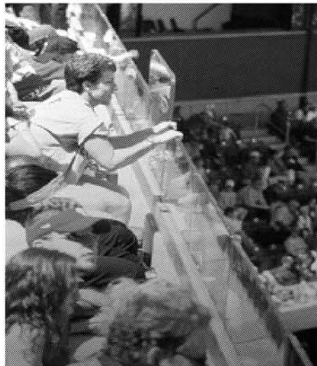
Figure 7 SentryGlas® Plus laminated glass balustrades, Citizen's Bank Park (Philadelphia, USA).
