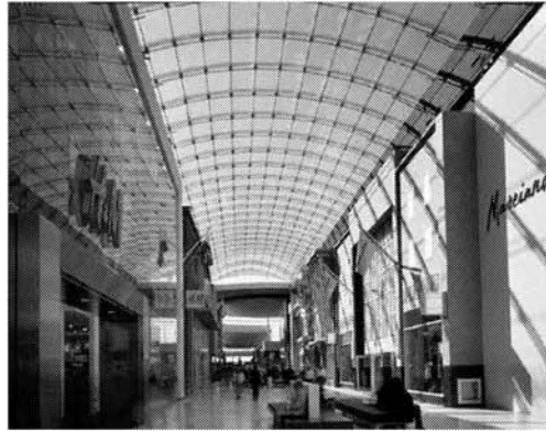
Figure 1 Planar™ | SentryGlas® Plus System in the Yorkdale Mall barrel vault roof (Toronto, Canada).
