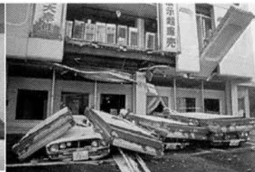
Falling wall panels Public Building, Kobe, 1995
