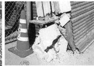
Destroyed column fixing San Francisco, 1989
