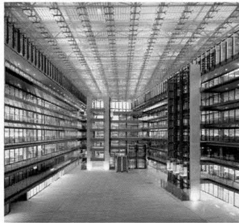
Figure 3 SentryGlas® Plus laminated glass roof structure of the Endesa Building (Madrid, Spain).
