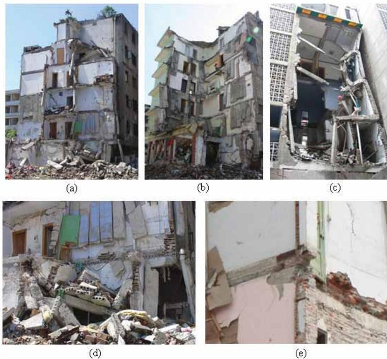
Figure 12. Damage of confined masonry buildings (a), (b), and (c) partial collapses, (d) collapse of simply supported hollow precast slabs, and (e) pullout failure of a beam
