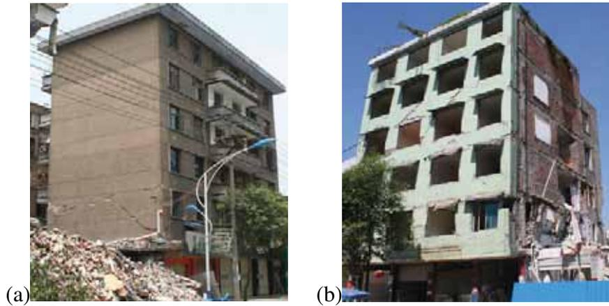
Figure 11. Damage to exterior masonry walls on top the first floors (a) extensive cracks and (b) out-of-plane dislocations
