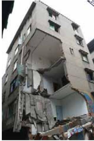
Figure 16. A partial collapsed 6-storey building due to collapse of load-bearing masonry walls at Mianyang city
