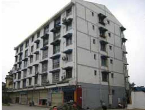
Figure 2. Typical confined masonry buildings in Sichuan
