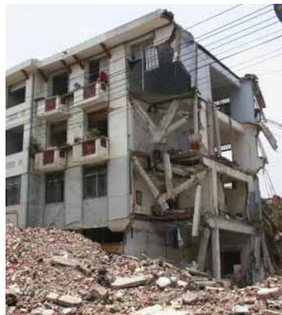
Figure 9. A 4-storey building without sufficient tie beams collapsed at Dujiangyan
